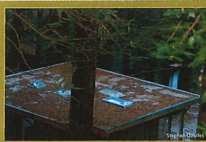
Photo 2. Minimal accumulation of vegetative debris accumulated on these dome-type skylights on this low-slope roof.
