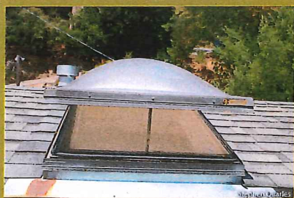
Photo 5. Operable skylights should be closed when a wildfire threatens. Similar to windows, they should incorporate a screen to resist the intrusion of embers (also good for insects!).
